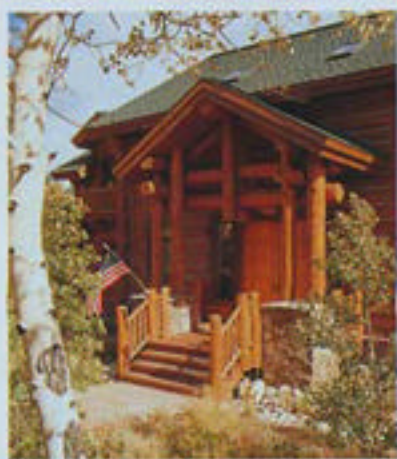
Top: The house was built in a grove of aspens at 10,000 feet elevation. The large-diameter logs are standing-dead Engelmann spruce shipped from British Columbia.
