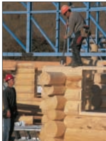
All beveling, arching and other visible log end details are sanded and properly finished. Ready for door and window installation.
