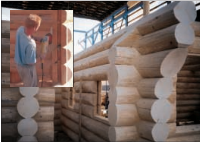
All beveling, arching and other visible log end details are sanded and properly finished. Ready for door and window installation.
