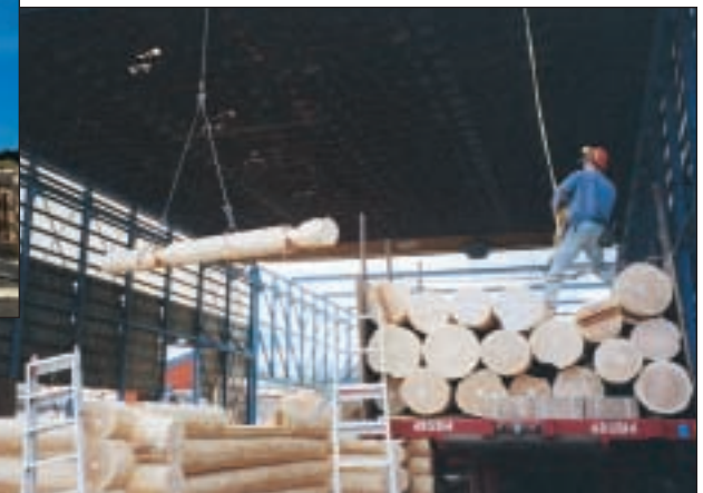
Upon completion of the log shell in our construction yard, the home is re-inspected for quality and it is number coded and loaded for shipment.
