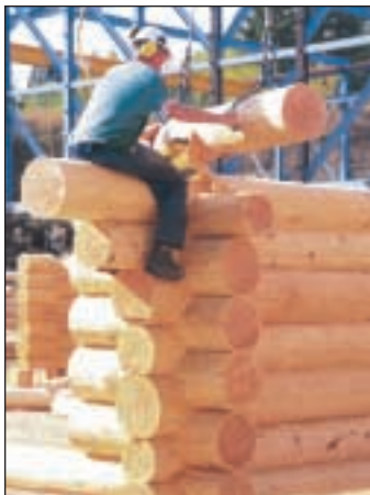
All beveling, arching and other visible log end details are sanded and properly finished. Ready for door and window installation.
