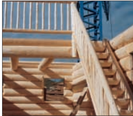
Mortise and Tenon Stair Detail
