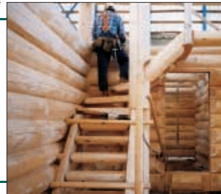
Mortise and Tenon Stair Detail
